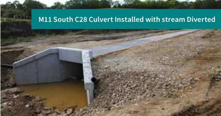
M11 South C28 Culvert Installed with stream Diverted
